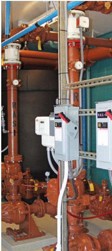
ABOVE: ITT Water & Wastewater – Flygt return activated sludge pumps and meters, and the non-potable water system tank (black, in back corner). RIGHT: Operator Dennis McCabe takes readings to monitor the aeration process.
